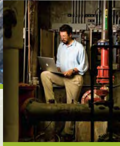
Professor Andrea Mammoli programs the digital controller, which automatically adjusts system parameters such as flow rates, fan operation, and building temperature as demand for power changes throughout the day.
