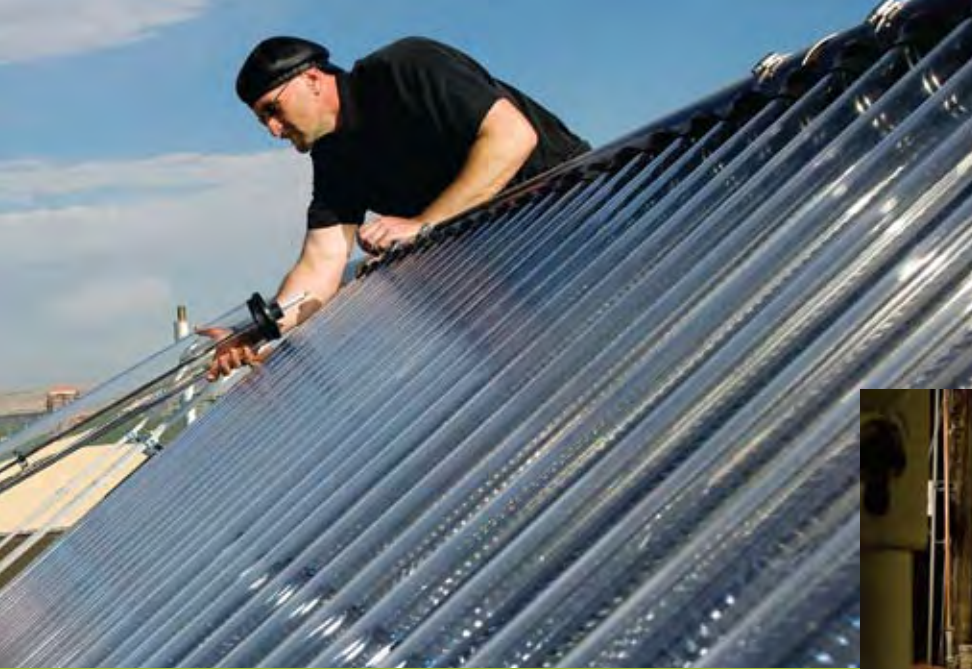
The ME solar team installs one of 640 state-of-the-art vacuum tube collectors on the roof of the Mechanical Engineering building.
