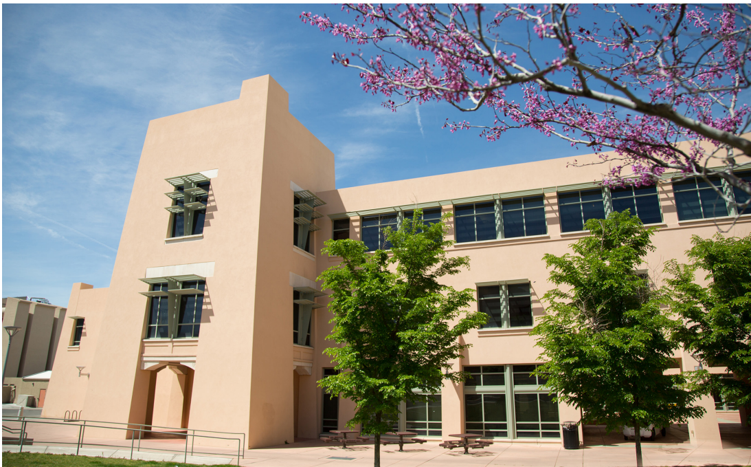
Centennial Engineering Center
